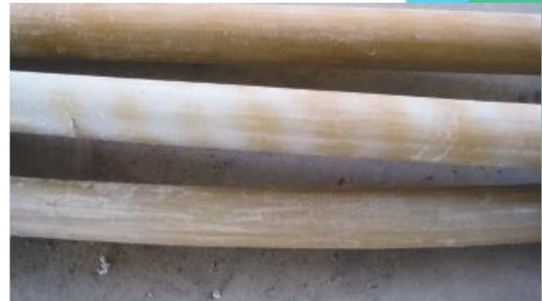
Figure 1: Discoloring process on cable insulation.
