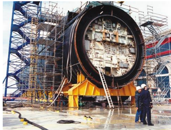
SSBN Redoutable Reactor Section
