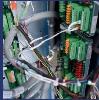
Instrumentation and Control
