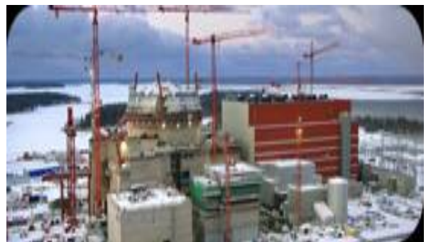
Usina Nuclear Olkiluoto 3 Cortesia AREVA
