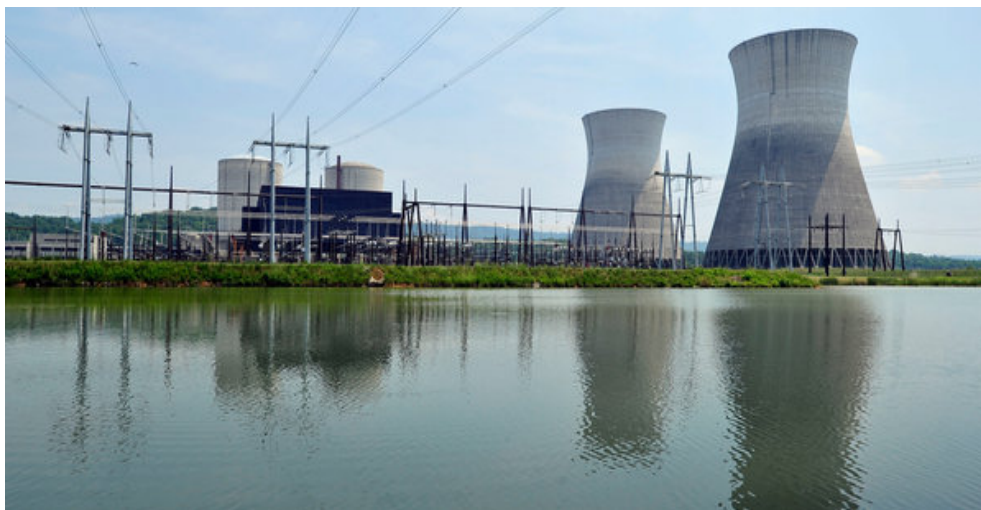
Bellefonte nuclear plant (The Tennessee Valley Authority's never-completed it, Alabama Foto : Eric Schultz/Associated Press
