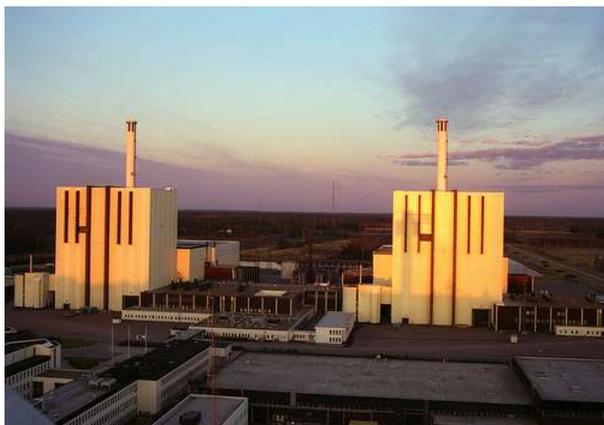
Central Nuclear de Ringhals (4 reatores- 3560MW)
