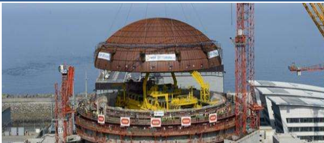
Flammanville – 3 – EPR 1600 MW (foto cortesia Edf)
