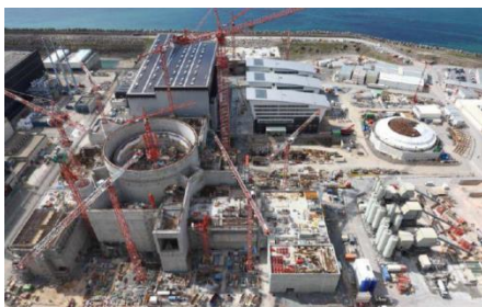
Flamanville-3 Construction began in 2007
