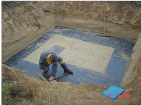
Studies on ageing of the bituminous membrane (Centre de la Manche)
