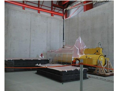
Remote handling system of a pilot reprocessing plant
