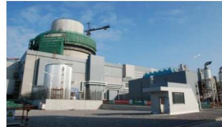
NI Capping 核岛土建封顶
