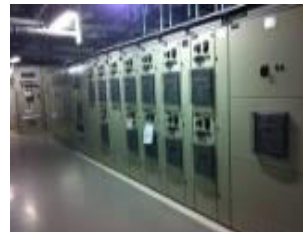
Electric, I&C Commissioning 电气、仪控调试
