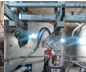
Half Tube Flushing Completed 半管冲洗完成
