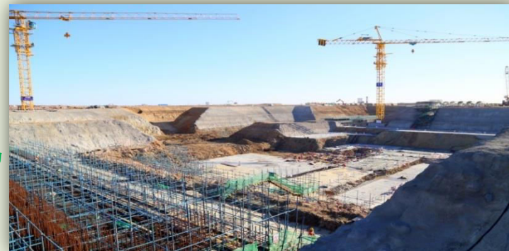
Under layer construction 垫层的施工
