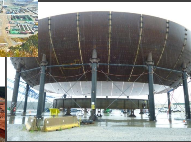
V.C. Summer 2 & 3 Containment Vessel Bottom Head
