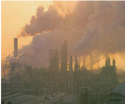
Flue gas Purification
