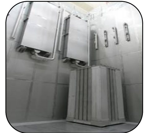
Passive Cooling Systems
