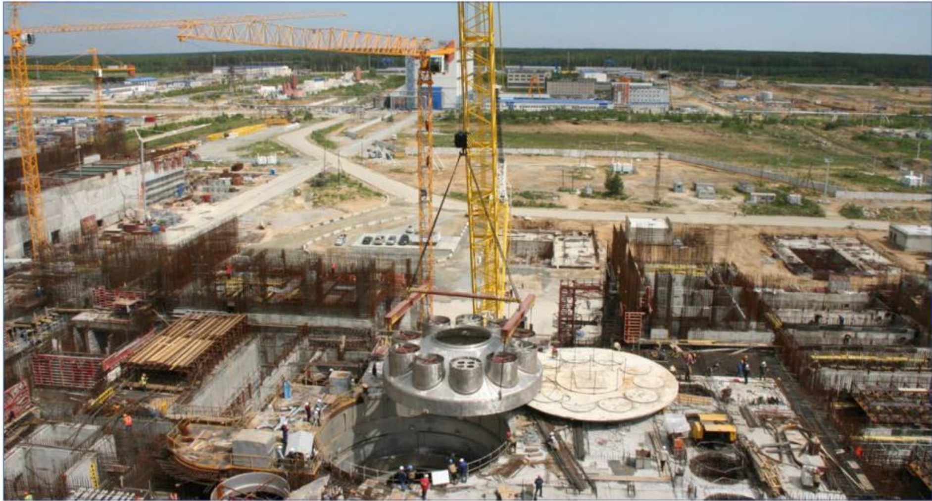
Construction Site of the BN-800 Fast Reactor at the Beloyarsk Nuclear Power Station, Russian Federation. (Photo: ROSATOM)
