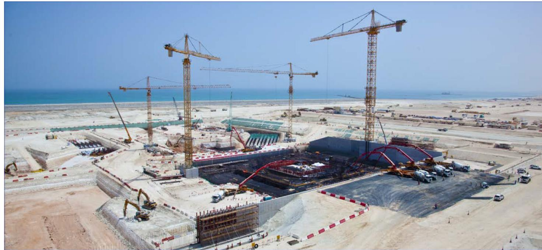
Construction Site of Unit 1, Barakah Nuclear Power Plant, UAE. (Photo: ENEC)
