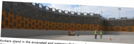
Workers stand in the excavated and waterproofed space for Vogtle 3's reactor building (Image: Southern)
